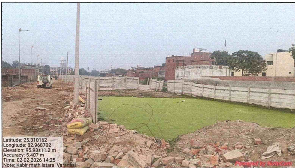
Photographs of joint committee inspection dated 02.02.26 at KABIRMATH, Lahartara.
